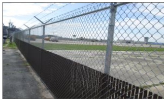
Obstruction Clearing & Fencing
